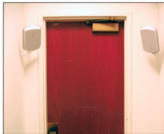
Files are automatically tracked as they enter or leave a department by the doorway.
