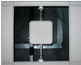
Files are automatically tracked as they arrive by sensors in the ceiling.
